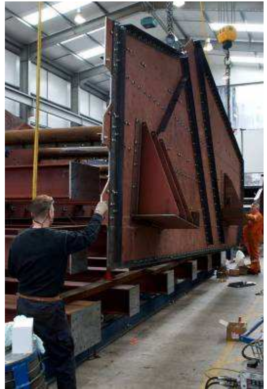
Second side plate being positioned
