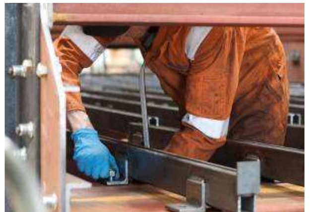
Deck members being installed
