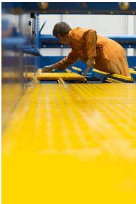
Deck panels being fitted
