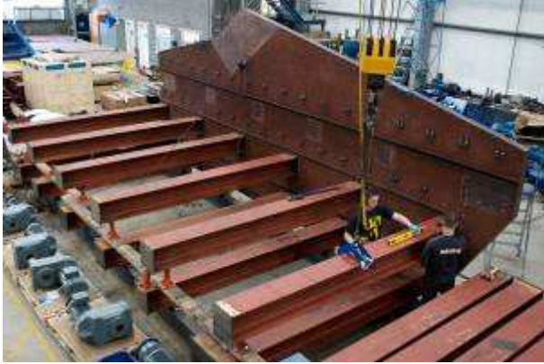
Cross members being positioned
