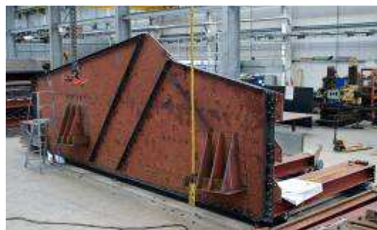
A side plate being attached to the cross members
