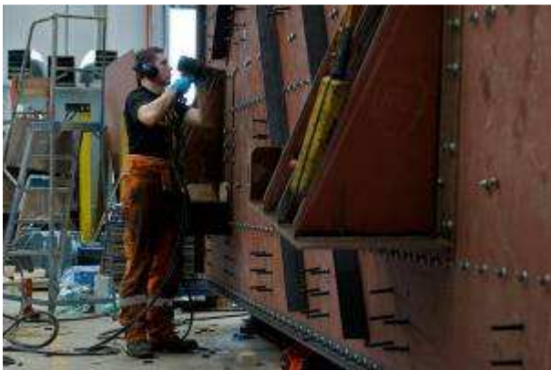
Side plate being Huck bolted in position
