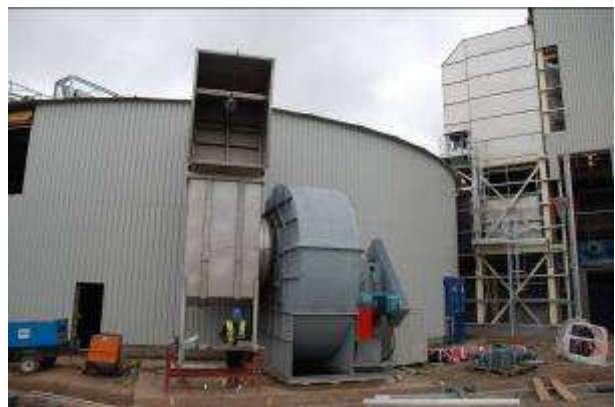
Germination fan for 350 te per batch GKV.
