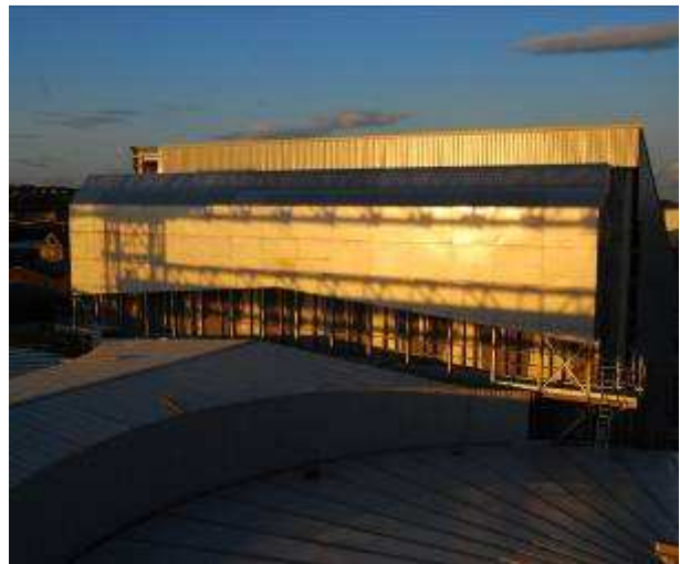
Heater house and air inlet shroud to heat exchanger.
