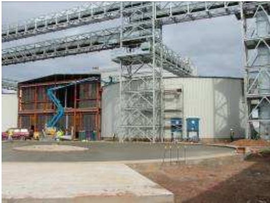
Feed and recovery conveyors to 2 x 350 te GKV's shown during construction.
