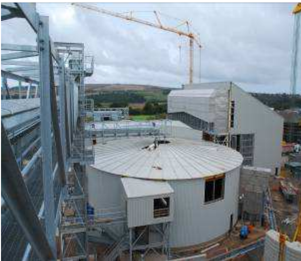
Two 350 te GKV's, heater house and feed System during construction.
