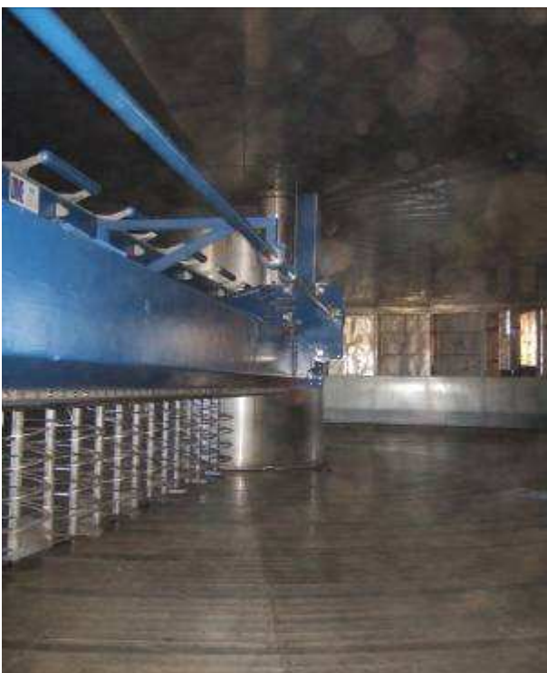
Inside 30m dia GKV with air on / off doors in background.
