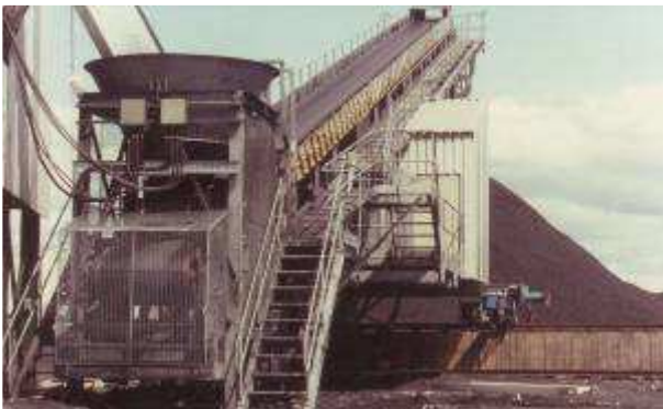
500 t.p.h. Radial Stacker delivering washed coal to stockpile
