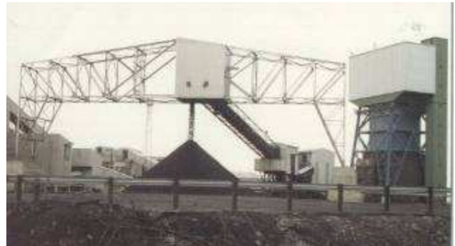
48 metre span stockout bridge delivering washed coal to stockpile.
