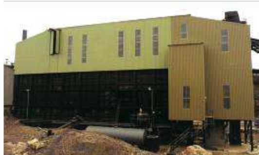
Graded Stone Storage Bunkers
