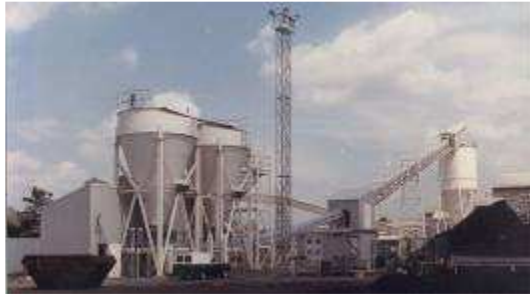
Coal Handling at a Cement Works (Showing Blending & Storage Silo's)
