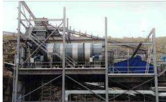
Limestone Washing Plant during construction.
