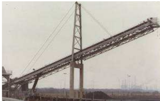
2800 t.p.h. Coal Stockout Conveyor
