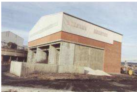
Filter Press House. Used for waste water clarification and the separation of Washery Tailings
