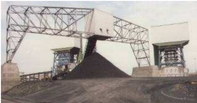
48 metre span stockout bridge delivering washed coal to stockpile.
