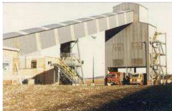
Lorry Loading Bunker
