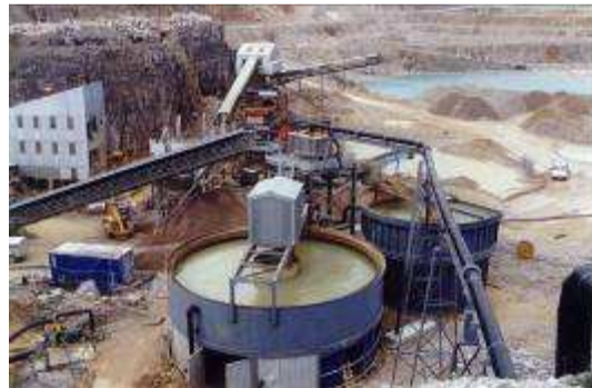
Two no. thickeners to handle fines from the Limestone Washing Plant.
