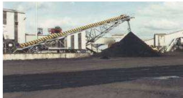
500 t.p.h. Radial Stacker delivering washed coal to stockpile
