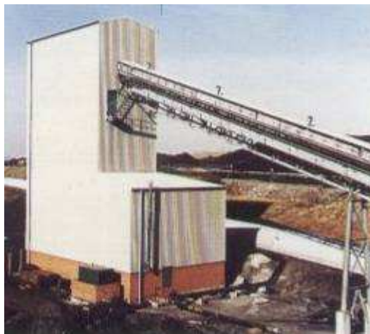
Mine Waste Handling System. Pumping -50mm Solids and Tailings over a distance of 2 km.
